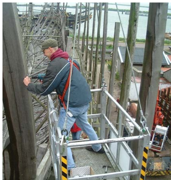
Fig.5. Placing landmarks as measuring points
